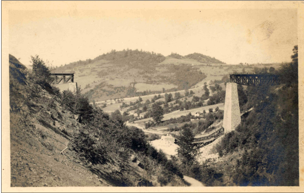
Picture of the damaged railway bridge near Volosianka.
